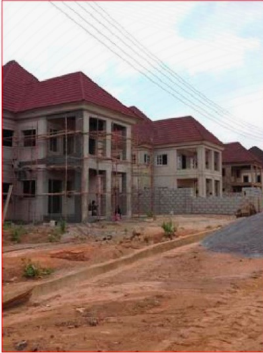
On Going Estate Development at Lokogoma District
